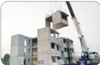
4. Prefabricated Sandwich Panel System
